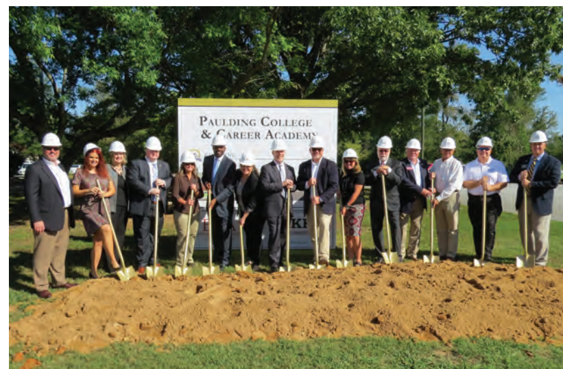
Above, Superintendent Dr. Brian Otott speaks at the ground-breaking event for the Paulding College & Career Academy.
